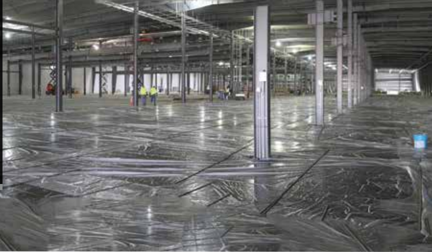
Viracon's facility expansion in Owatonna, Minn. | Photo Credit: Viracon Inc.
