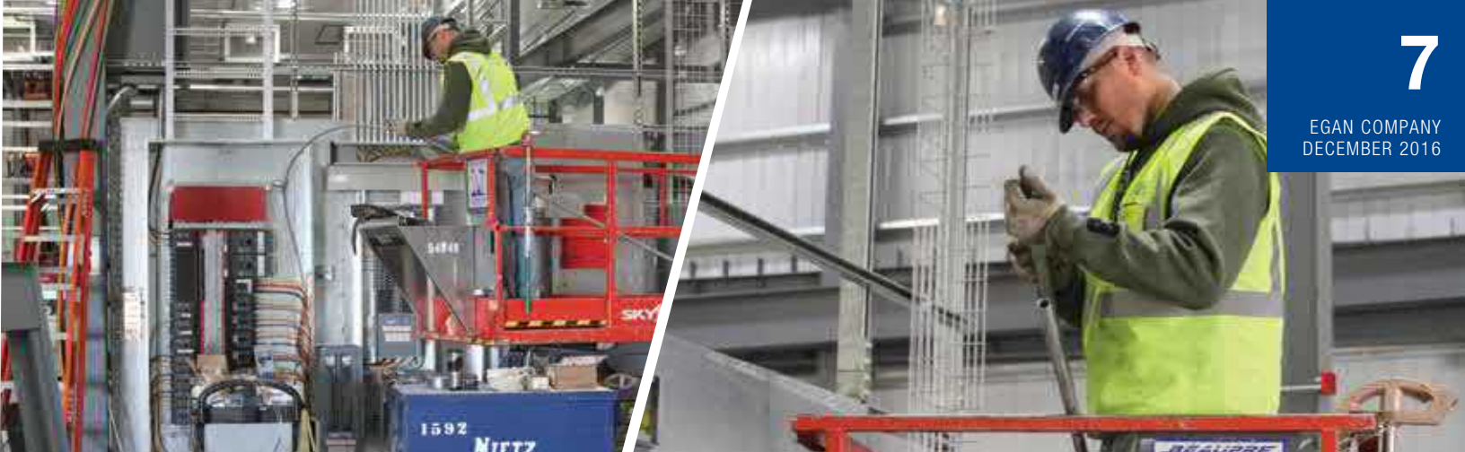
Viracon's facility expansion in Owatonna, Minn. | Photo Credit: Viracon Inc.
