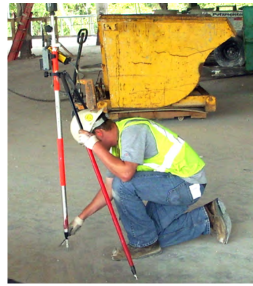
Above: Mike Gerde (Egan Company Sheet Metal worker) locates and marks the points on the structure.
